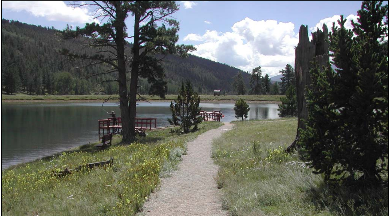
Shuree Pond (NECF-2009-010) parking lot and trails were hardened and graded to keep erosion from entering the lake.
