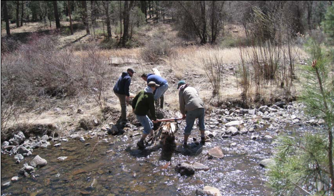
HSP funds (SWFG-2009-003) were leveraged those of the NM Environment Department to place trees into Black Canyon Creek in order to create pools for trout in the Gila National Forest near Mimbres. Volunteers from NM State University provided the muscle. Photo courtesy of Tawnya Brummett, USFS.
