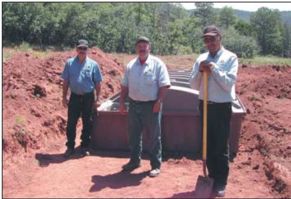
Department of Game and Fish construction crewmembers, from left, Jon Chafins, Bill Taylor and Juan Chavez did the hard part of installing a guzzler that captures rain and snow for use by wildlife on the Bluebird Wildlife Management Area.
